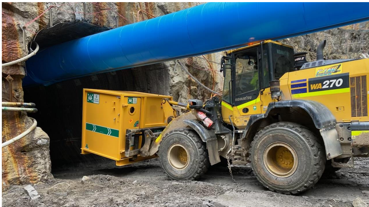
Figure 1 Installing a refuge chamber
